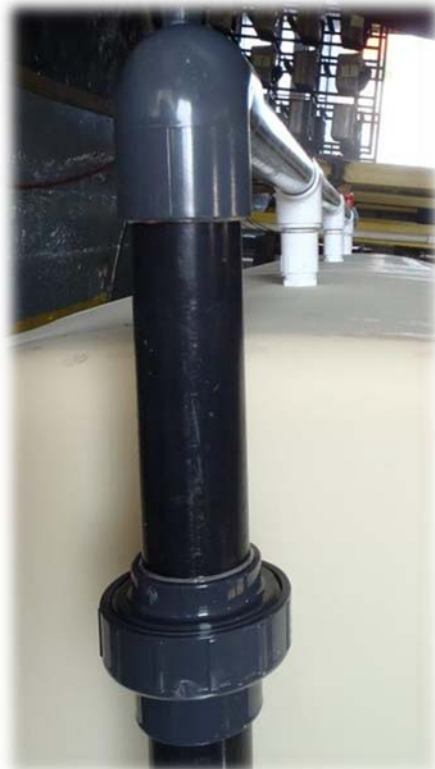
2" Snap-On Fill Line Supports
